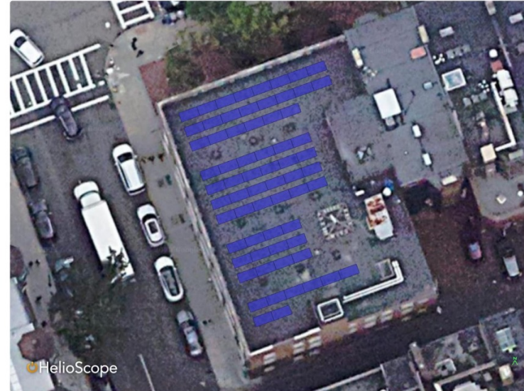
Figure 3. Location of on-site solar system at [redacted] developed through HeliScope.
